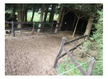
As the final step the stones were covered with a 5 cm mulch top layer to protect the horses hooves.
