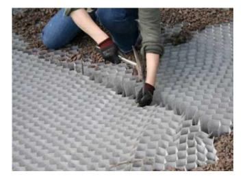
The grids were first extended side by side and were temporarily fixed with pegs, before the adjacent cells were tuckered together. After filling the cells, the pegs may be removed, or hammered down to the same level as the grid.
