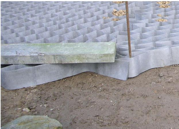
*Ensure the grid is in contact with the ground before filling, to prevent lifting of the grid.*
