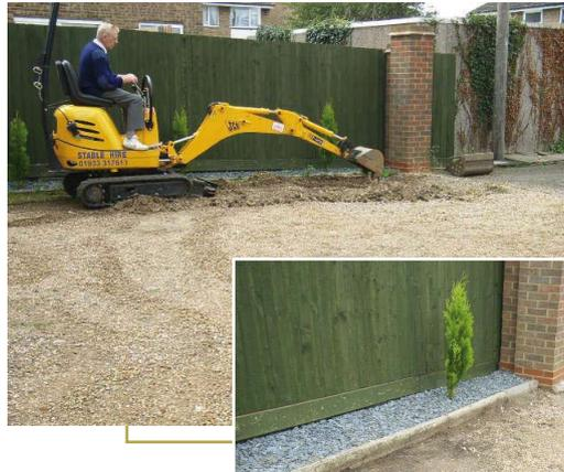
To relay the drive with DuPont™ Ground Grid, the ground was prepared first by removing approximately 65mm with a mechanical digger.
